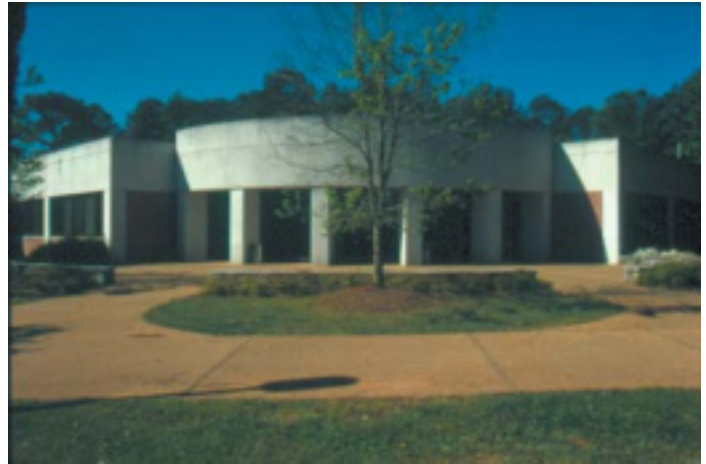
Technology Building at Clayton College & State University, one of seven campus buildings served by the central plant's Aerco boilers.
