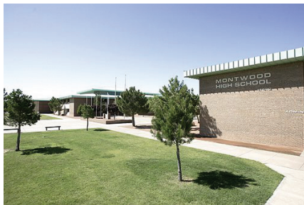
El Paso's Montwood HS suffered from air in its heating system for over a decade
